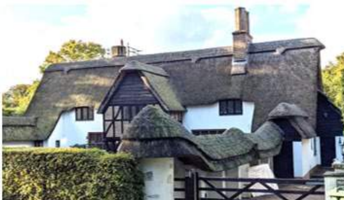
Blair Imrie houses Old Avenue Conservation Area West Byfleet built 1911 to 1913
